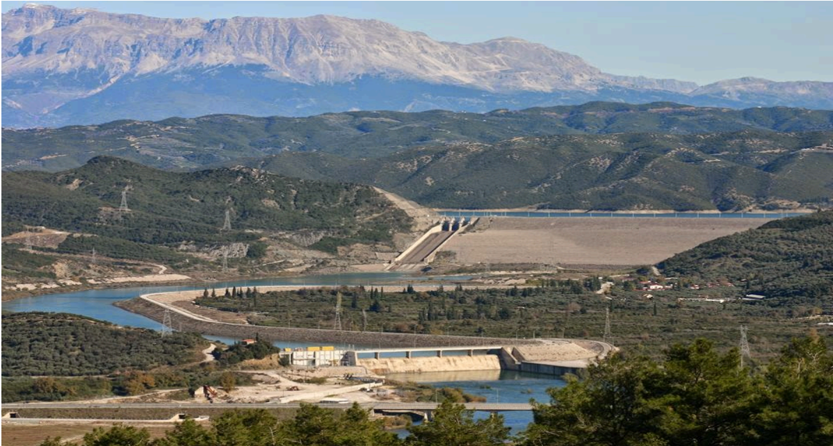
Picture 2-12 Hydroelectric dams of Pournari I and II, at Arta Greece.
