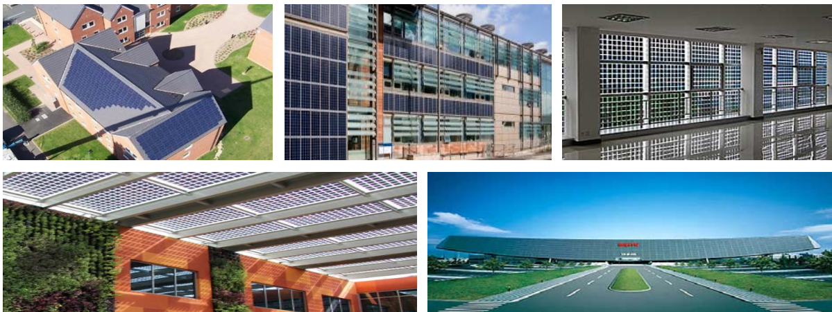
Picture 2-9 Applications of building integrated PVs at rooftops, building facade, windows, sunshades and the gorgeous solar arc at Sanyo's semiconductor factory in Gifu, Japan (bottom and right).
