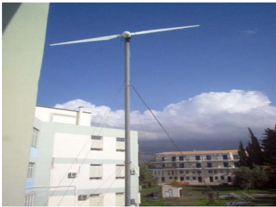
Picture 2-4 A whisper type wind turbine on the roof of Renewable Energy Systems & Sources Laboratory roof, Technological Educational Institute of Western Greece, Patra.
