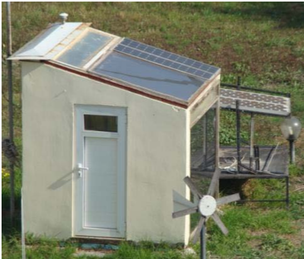
Figure 1-8 Intelligent Energy Building (test cell), at Renewable Energy Sources & Systems Laboratory, of technological educational institute of western Greece, Patra.
