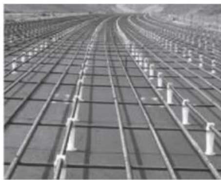
Reinforcement ready for concrete
