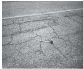
Block cracking
