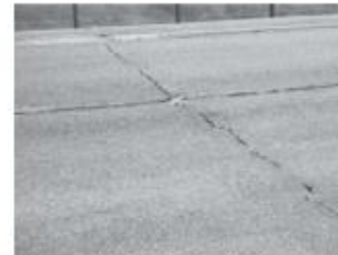
Reflective cracking
