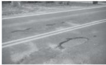
Delamination
