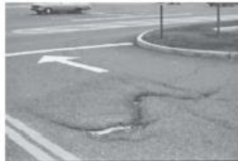
Slippage crack
